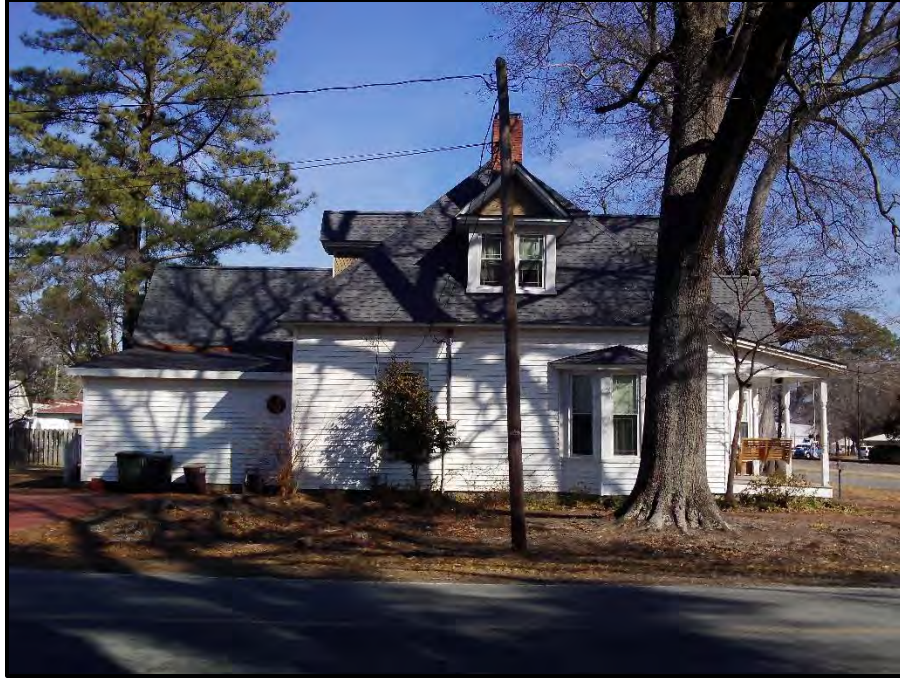
Figure 5. Claude Bandy House (JT1125), View Looking Northeast.
