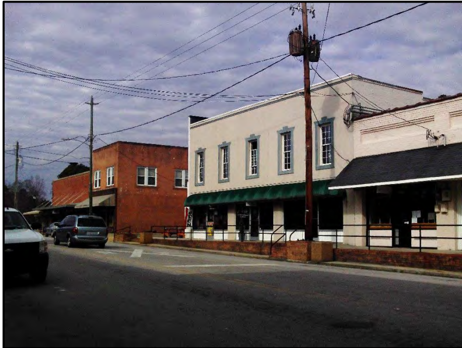
Figure 20. Streetscape of S. Main Street at Intersection of E. Wellons Street, View Looking North.
