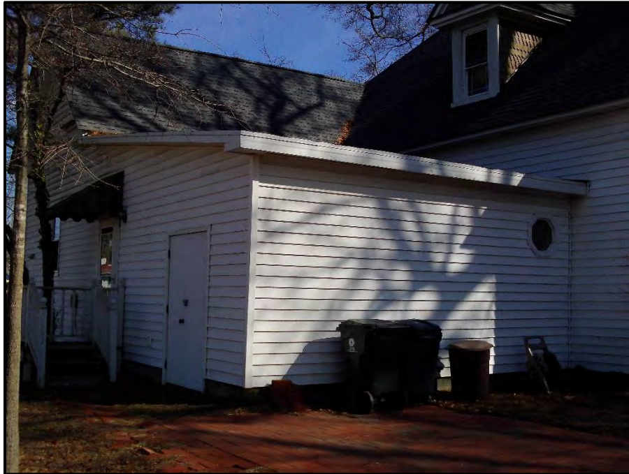
Figure 13. Detail of Shed-Roofed Wing off EII, View Looking East.
