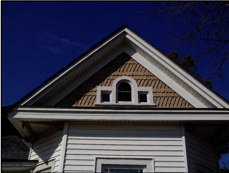
Figure 8. Detail of Patterned Shingles in Gable of Projecting Bay, View Looking Northwest.
