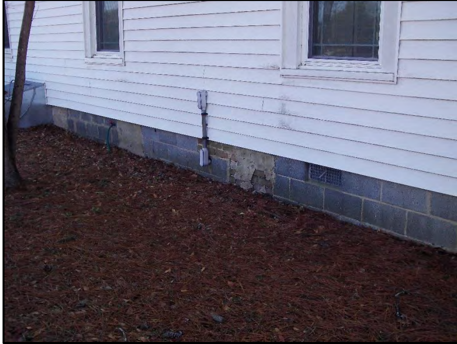
Figure 12. Detail of Foundation, View Looking South.
