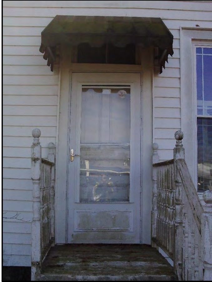
Figure 11. Detail of Rear Entry Door, View Looking Southeast.
